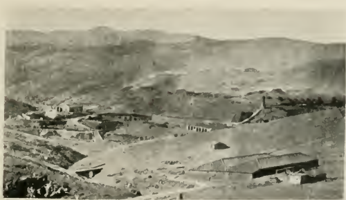
CEMENTATION VATS, HUELVA.
